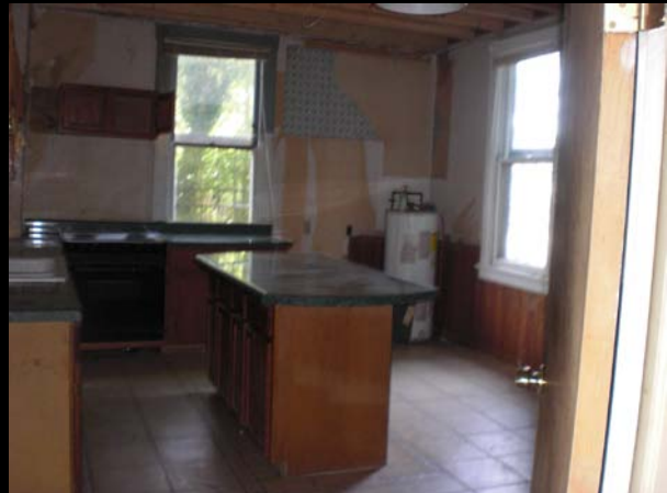
KITCHEN DONE ON ONE SIDE
